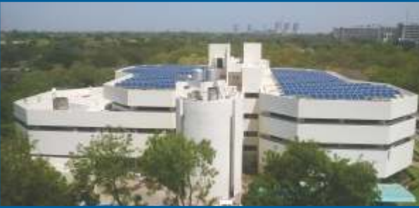
Installed Capacity- 100KWp Location- Gandhinagar
